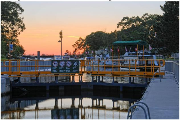
As a part of these important investments, the lock gates at Fenelon Falls Lock 34 have been scheduled for painting. Painting and routine maintenance helps to extend the lifespan of lock gates by protecting against rusting, corrosion, and natural wear.
