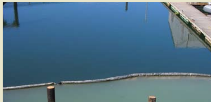
A marine silt fence was maintained throughout construction to reduce siltation
