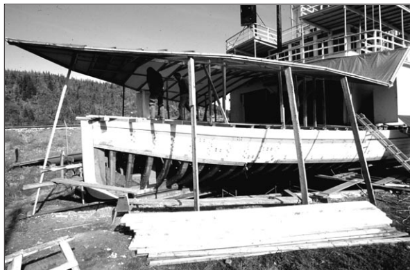
Stabilization of the hull
